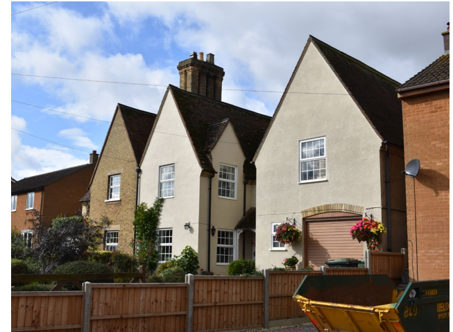
Figure 19: Acute triangular gable rooflines.
