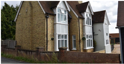
Low brick wall boundary
