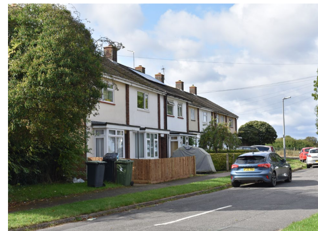
Figure 09: View down West Way, short cul-de-sac off Blunham Road.
