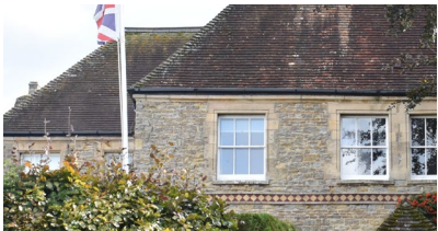
Coursed limestone rubble with ashlar dressings
