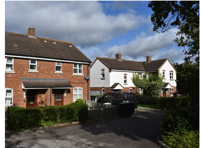
Figure 17: Two storey dwellings, typical of Moggerhanger.
