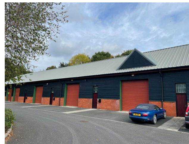
Figure 33: External positive example of light industrial units.
