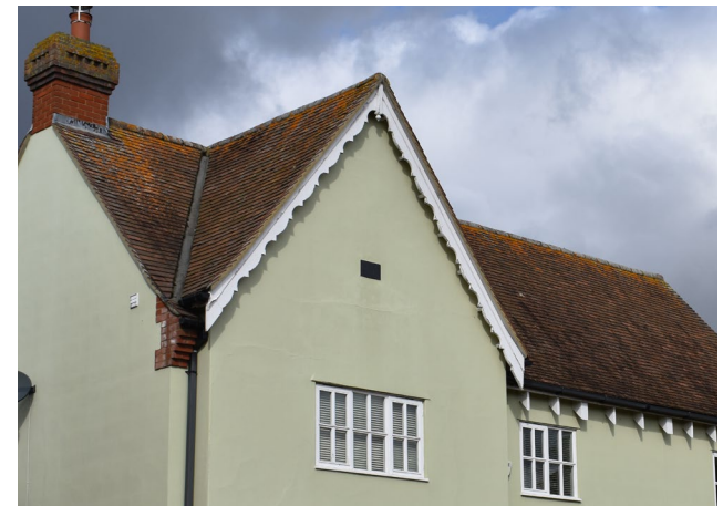
Figure 20: Triangular gable with decorative fascia board.
