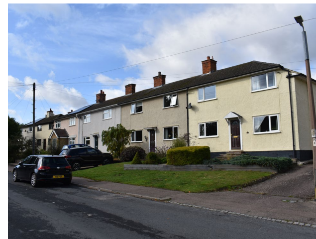
Figure 08: Short terrace on Blunham Road.
